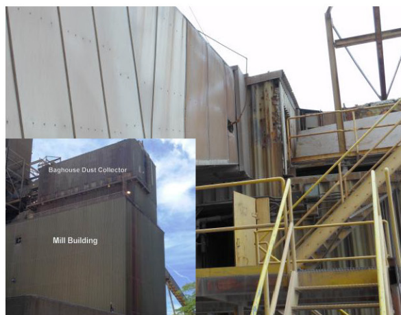
Deteriorating Kiln/Raw Mill Baghouse
